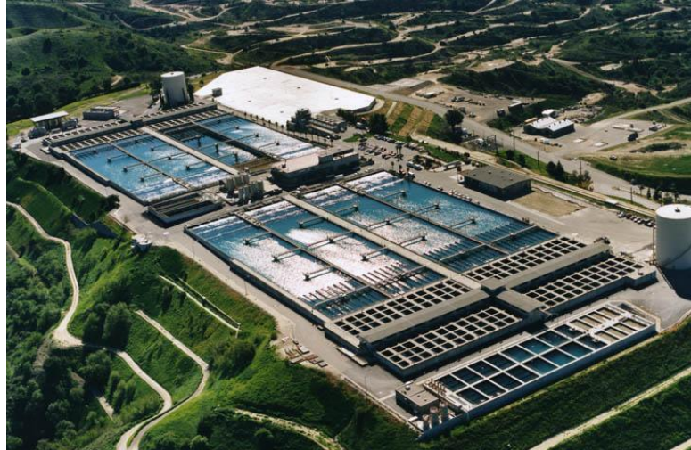
Figure B- 5. Diemer Water Treatment Plant, Yorba Linda
